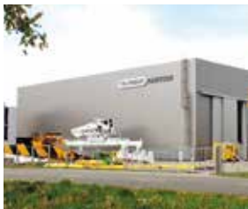
Offshore Cranes Gdynia, Poland
