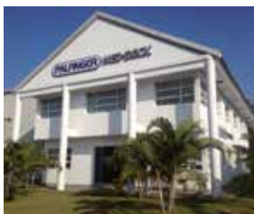
Launch and Recovery Systems Hanoi, Vietnam
